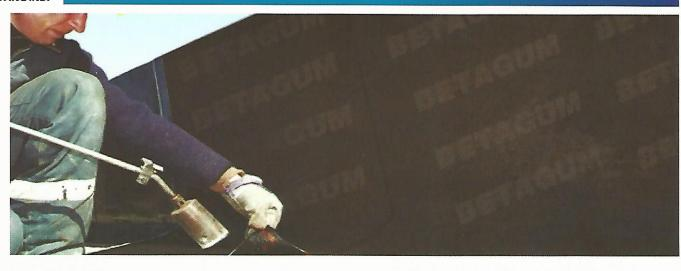
**BETABOARD** is a tough semi-flexible, rot-proof, durable pre-molded bitumen based board suitable for a variety of applications in below or above ground waterproofing as well as roofing, parking, bridge decks, wet areas, planters, pools, fountains and civil works.
