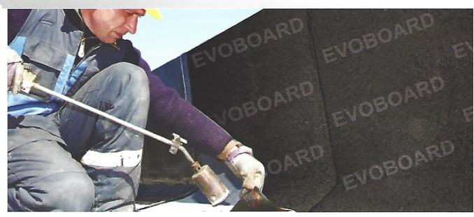
EVOBOARD is a tough semi-flexible, rot-proof, durable pre-molded bitumen based board suitable for a variety of applications in below or above ground waterproofing as well as roofing, parking, bridge decks, wet areas, planters, pools, fountains and civil works.
